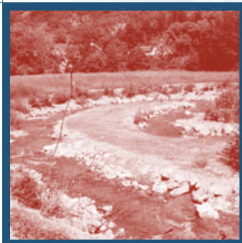
Naturelike bypass channel, Austria © BOKU
