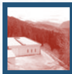
La Zour drinking water power plant in Switzerland © MHyLab
