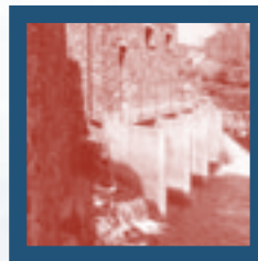
Powerhouse dressed in local material © IT Power
